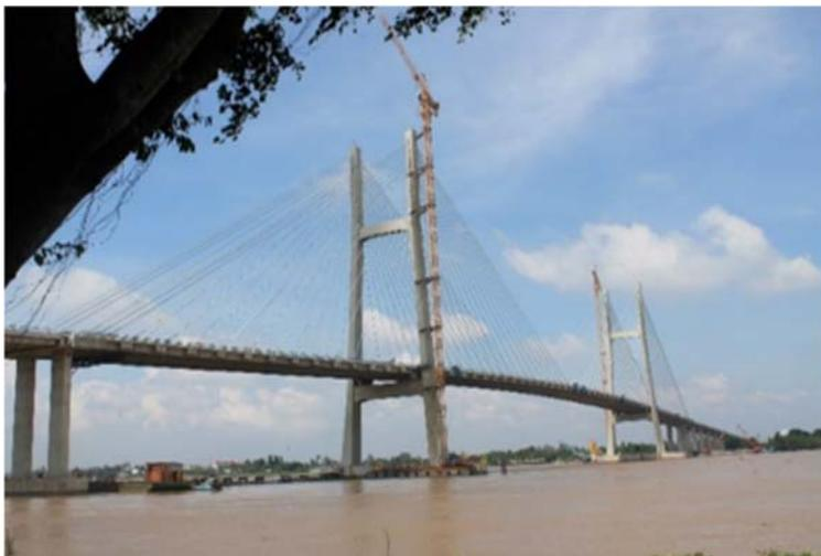
*The Cao Lanh bridge, a cable-stayed bridge, under construction over the Tien River at Cao Lanh, Dong Thap Province, Viet Nam. It is one of three components of the project.*
